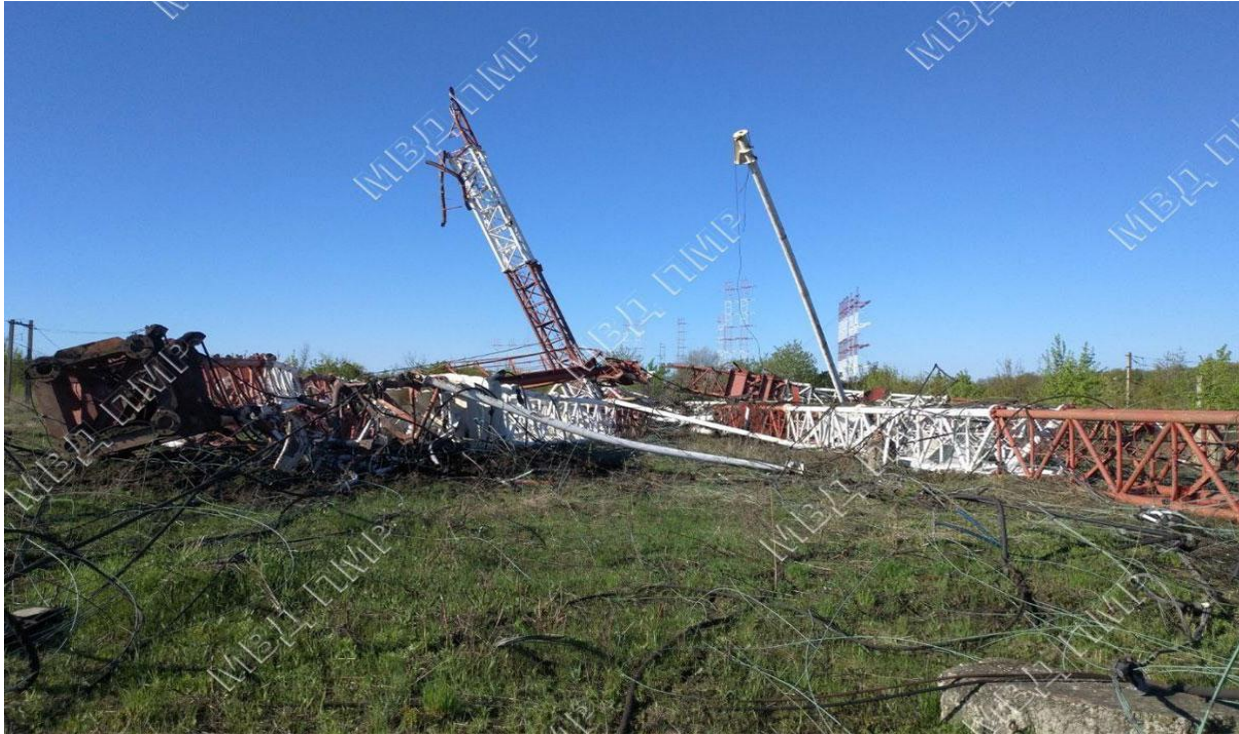
Fig 2. Radio transmission towers at Maiak after the attack. April 2022.
